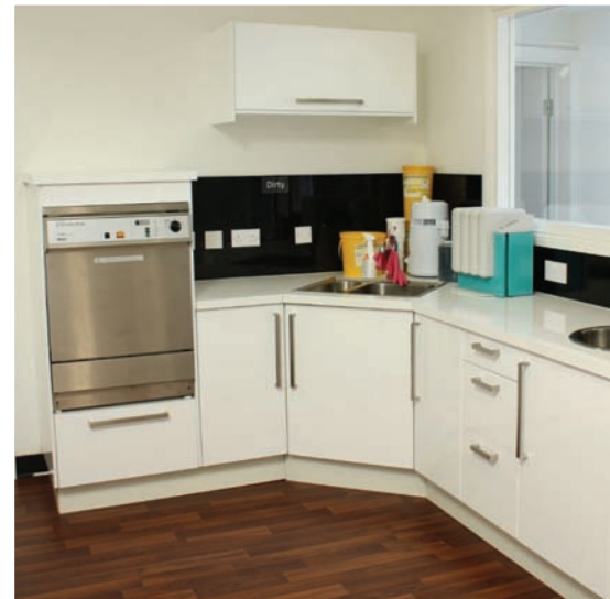
Part of the sterilisation room (dirty side)
